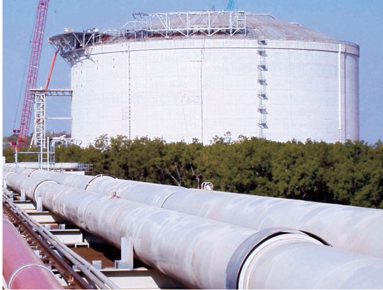
Darwin LNG liquefaction facility in Northern Territory, Australia, including Chart vacuum-insulated pipe and vacuum-insulated pipe riser modules for large storage tanks
